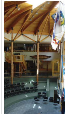
Trees harvested from the construction site used for structure and roof.
