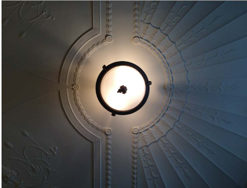
Figure 6 – Interior elements: Ceilings
