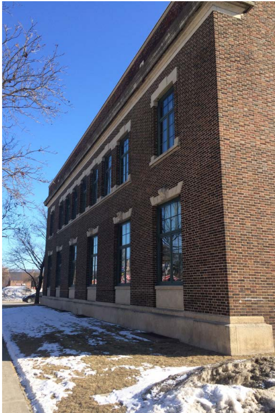
Figure 3 – Side View: Laird Norton Building, along Johnson St. Winona, Minnesota
