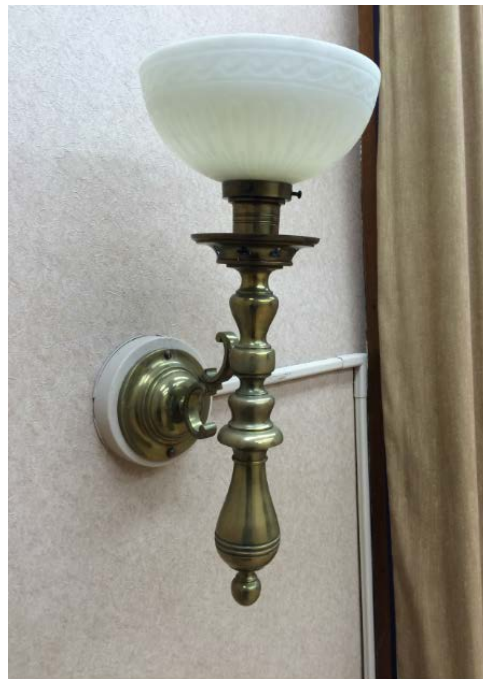
Figure 7 – Interior elements: Light fixtures
