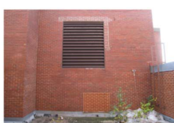
MEC roof and exterior wall
