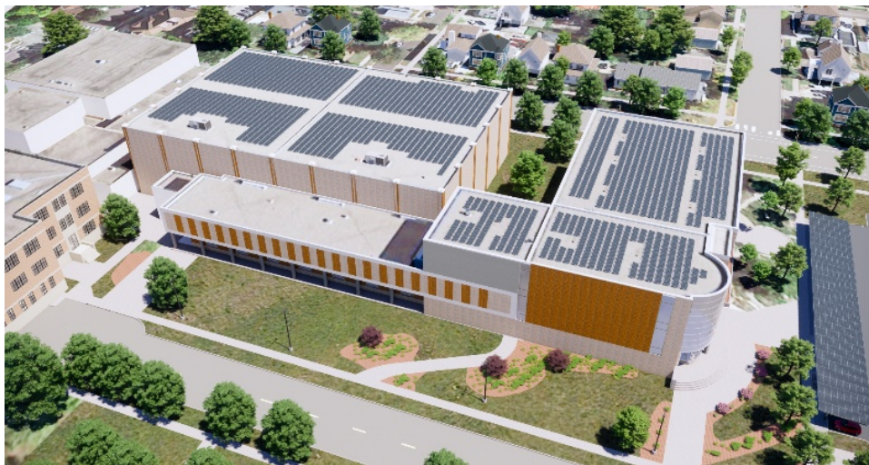
Campus view of the solar rooftops
