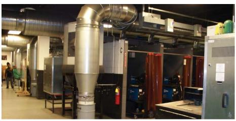
Welding shop fume recovery system takes all of the smoke and particulate out of the air putting the conditioned air back into the shop instead of 100% exhaust that is typical in welding shops.
