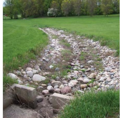
Water-way designed to slow water to control erosion.
