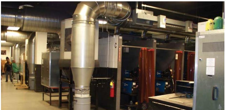
Welding shop fume recovery system takes all of the smoke and particulate out of the air putting the conditioned air back into the shop instead of 100% exhaust that is typical in welding shops.
