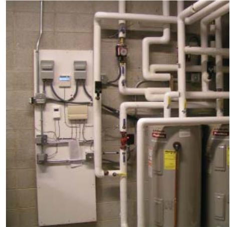
Heat transfer piping for roof-top solar panel system.
