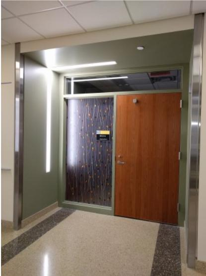
*Decorative film can be installed on sidelights to provide partial views and light transfer while also reducing distractions within the classroom.*
