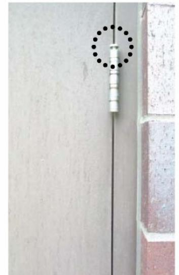
*This exterior hinge pin could be easily removed to gain access.*
