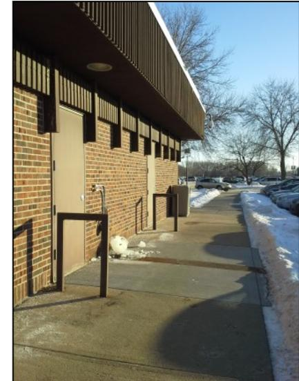
*If emergency exit doors must open onto a primary pedestrian route, provide protective railings within the door swing area.*
